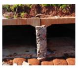
by Lancer Communities. 'Aspire' at Evanston South involves the installation of Gabions along the sides of a creek. We also designed and constructed Gabion facades to cover the concrete culverts to help add to the asthetic look of the finished project.
