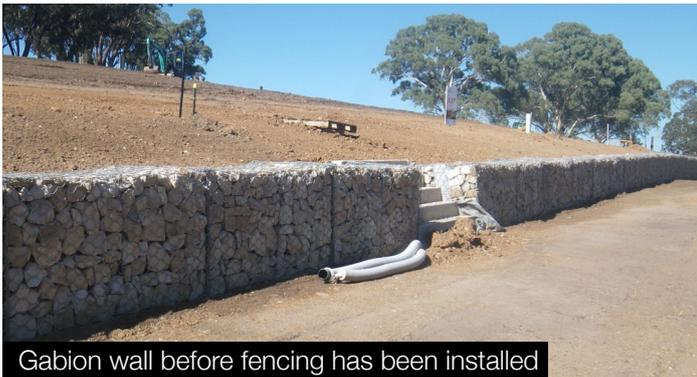
Gabion wall before fencing has been installed
