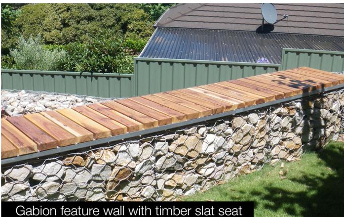
Gabion feature wall with timber slat seat
