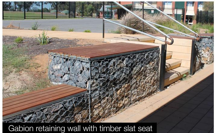
Gabion retaining wall with timber slat seat
