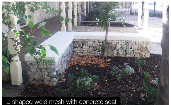
L-shaped weld mesh with concrete seat
